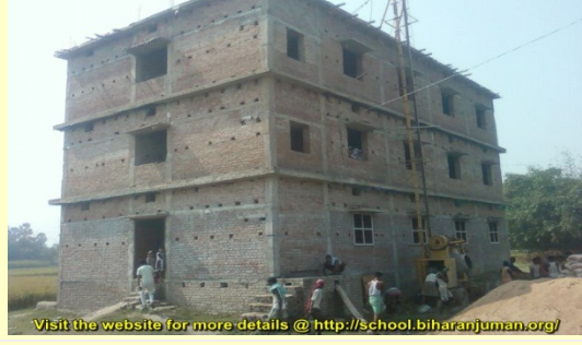
RAHBAR-e-Banat School and Madrasa, for holistic education & guidance For Girls of weaker sections: Hostel Bldg's 3rd Floor roof east on 29-10-2011
