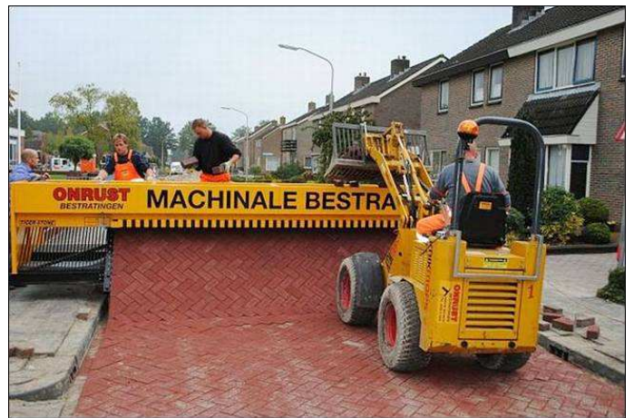
Road making machine by bricks
